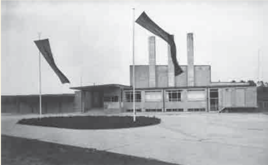
Hannes Meyer, Hans Wittwer and the Dessau Bauhaus building department: General German Trades Union school in Bernau, near Berlin, 1928-30. Meyer and Wittwer made the three chimneys of the oil-firing system the dominant motif of the school's entrance, leading one pupil to describe it as an "education factory". On the right, a loading ramp; left, garages.*
